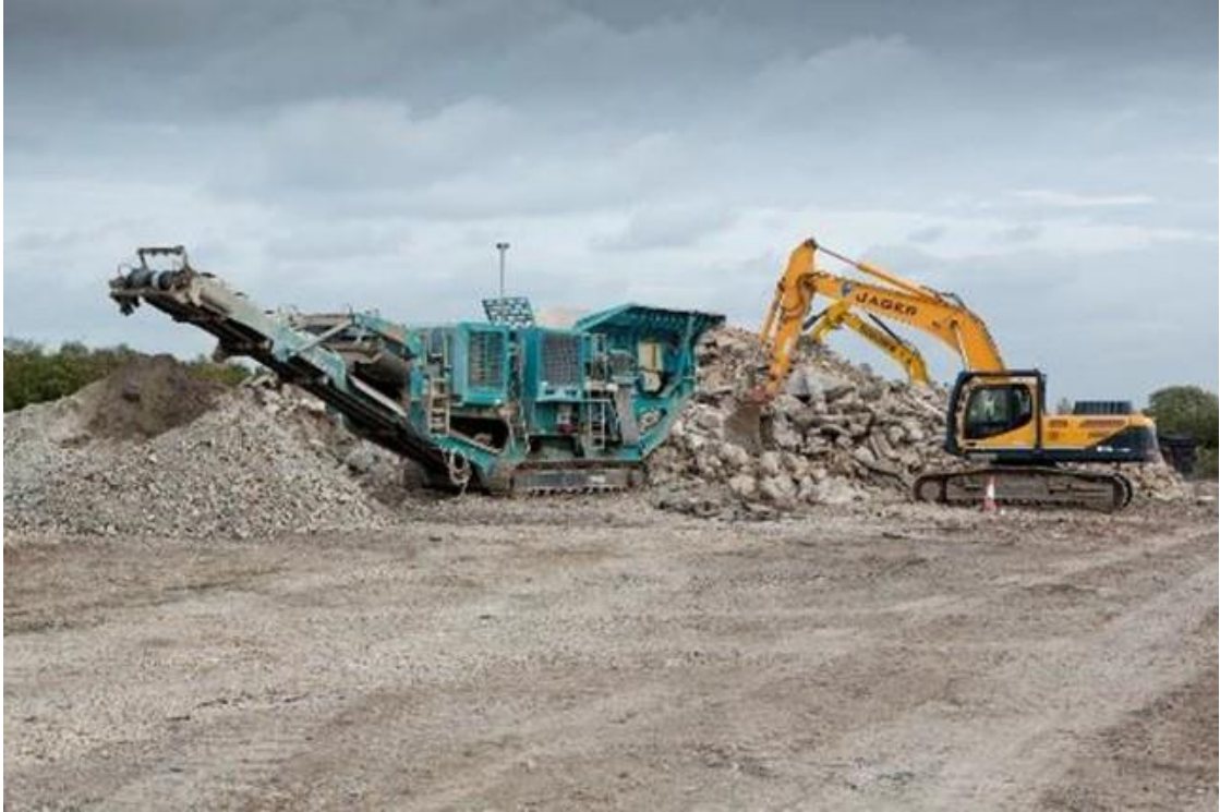
Figure 3: Example of site-based crusher arrangement (Old Oak Common Crossrail Depot)
