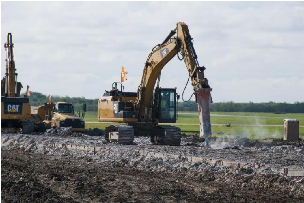
Figure 2: Typical concrete pavement demolition operation using percussive hammer breakers
